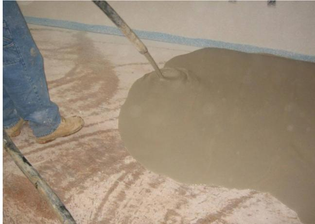
Gypsum Concrete is commonly used as a floor underlayment in wood-frame multi-family construction for fire ratings, sound reduction, radiant heating and smooth surface. The basic mixture includes gypsum, portland cement, sand and water. It installs by pumping a very low-viscosity mixture of water and underlayment on the wood subfloor to a desired thickness, commonly 3/4-inch. When dry, a very smooth surface is left for the installation of finished flooring.
